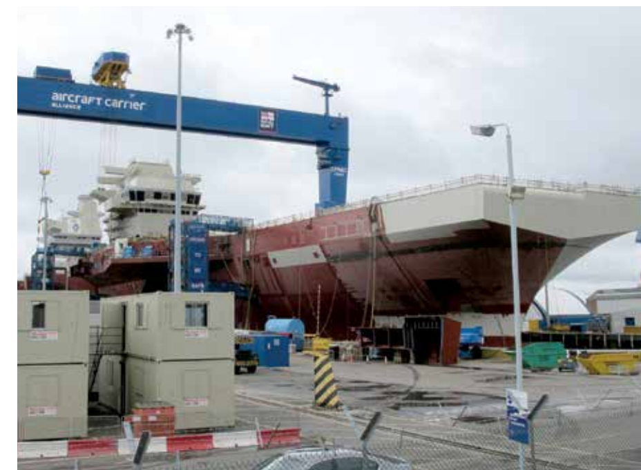
The part-completed Queen Elizabeth at Rosyth shipyard
